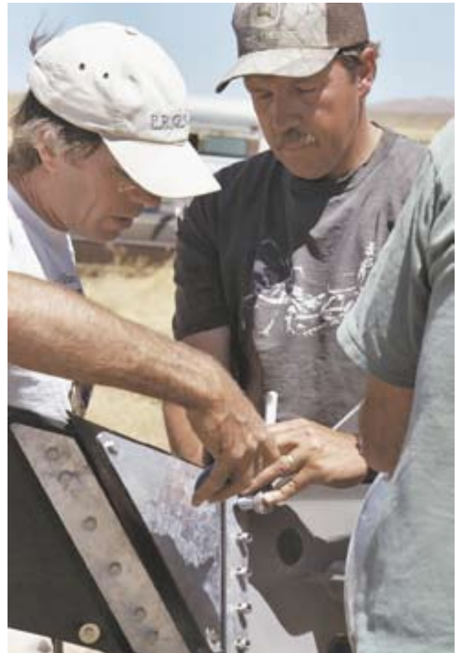
Installer Chris Worcester, and owner Paul Thomas attach blades to the Proven's downwind hub.
