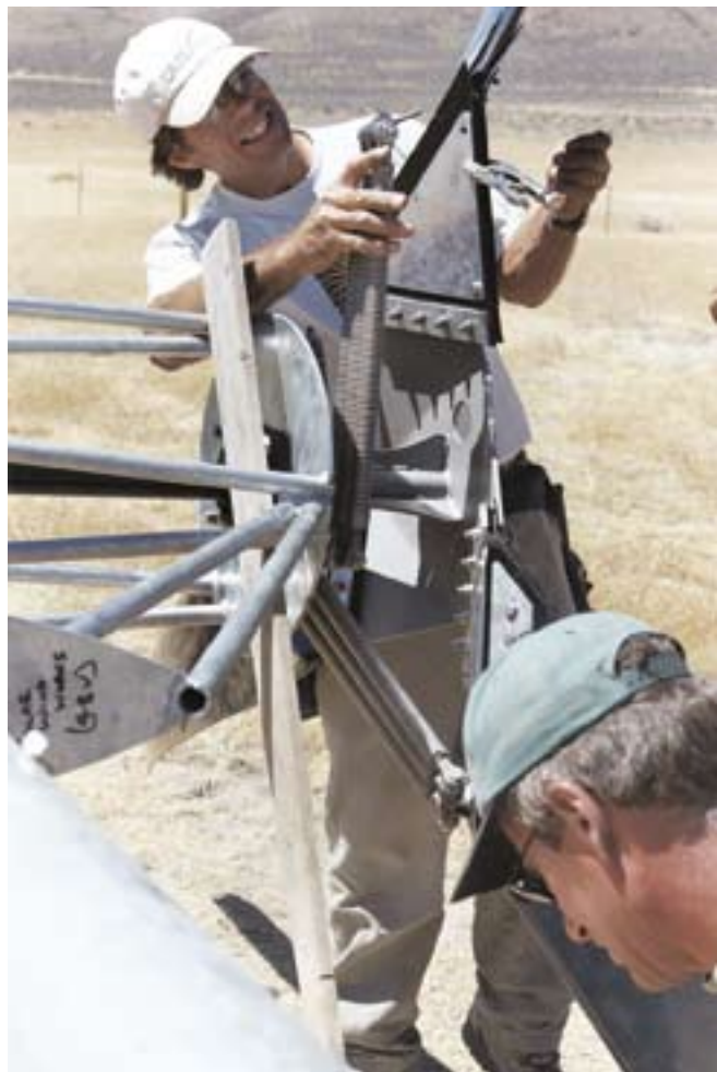
Chris attaches a spring pack which tensions the blade during high-wind governing.
